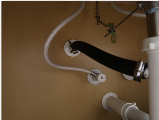
Primary Drain Line
