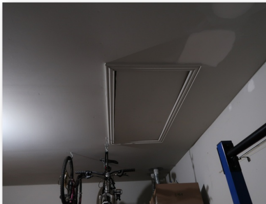
Attic/Roof Structure Ventilation Type :Box Vent, Soffit Vent
