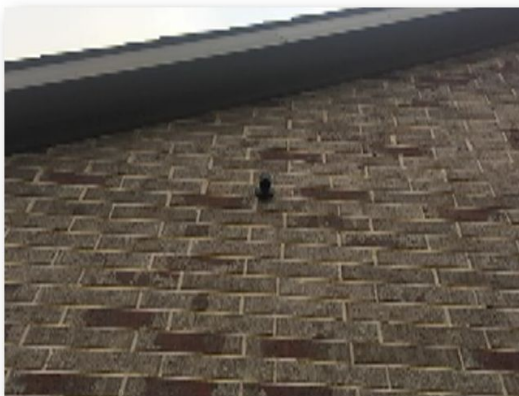
Secondary Drain Line
